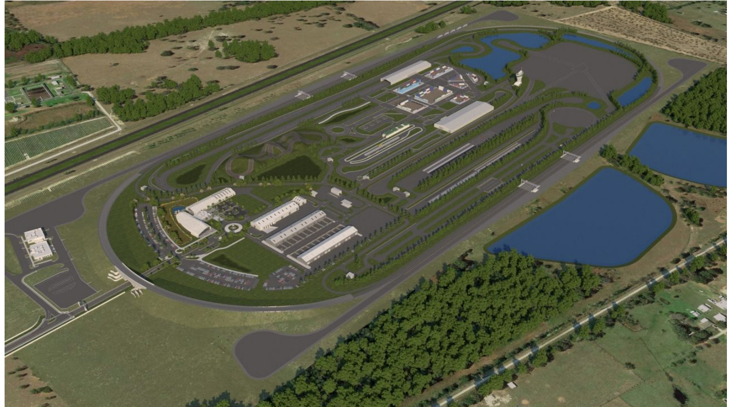
SunTrax Toll and CAV Test Facility, Lakeland FL
